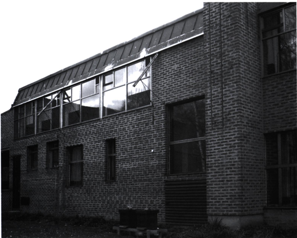
Figure 11. Church of St Mark, Björkhagen, Stockholm, 1956-64. Architect: Sigurd Lewerentz. Eastern façade. In some of the windows, the glass panel is fixed directly onto the wall. Photograph by the author.
